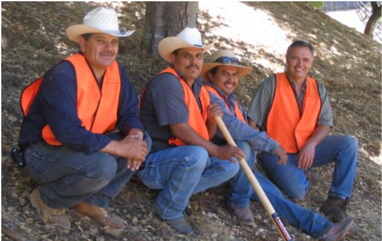
Crew working on sprinkler valve repair.
